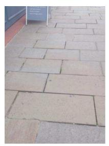
Recent inspections of the paving on Reigate High St and Church St have revealed several loose slabs and a large amount of missing cement between the slabs. The problem is particularly acute on the North side but isolated patches exist on the South side.
